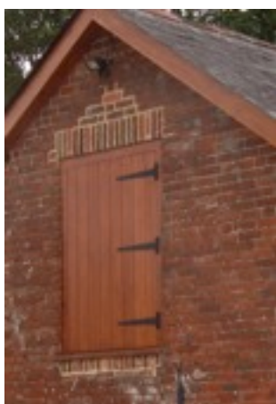
Poor brickwork repair
